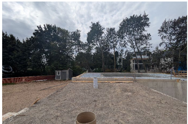
View of the abutting property to the west from the location of the balcony
