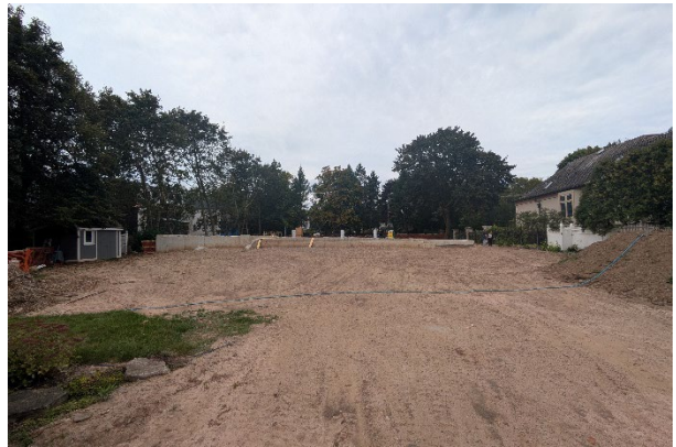
View of the dwelling under construction
