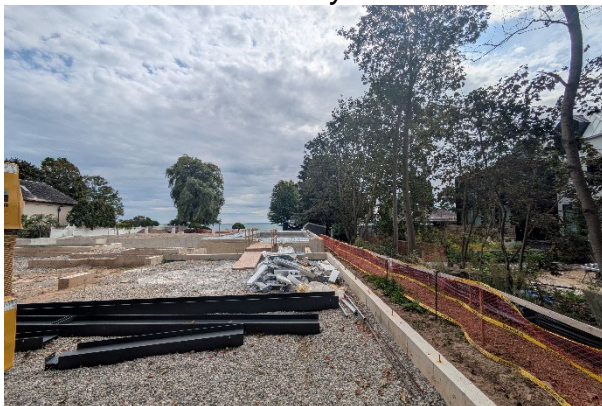
View of the dwelling under construction and the abutting property to the west
