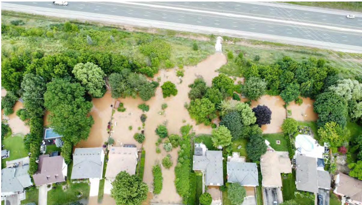
Hwy. 407 embankment failure partly blamed for 'devastating' flood impacting Burlington, Ont., homes: mayor. Samantha Beattie, CBC News, July 18, 2024
