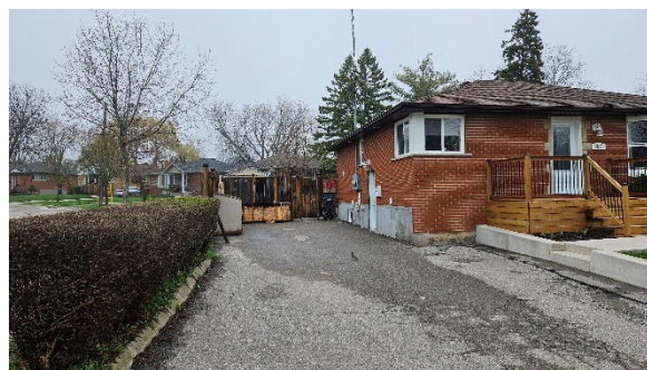
Abutting property at 1483 Fisher Avenue (at corner of Fisher Place)
