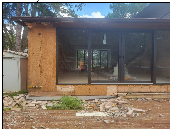
View of the addition
