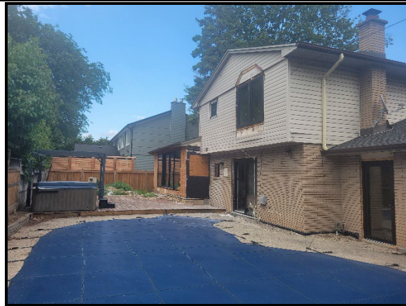
View from the rear yard
