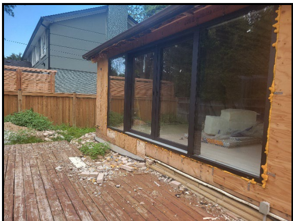
View of the addition and the northerly abutting property beyond
