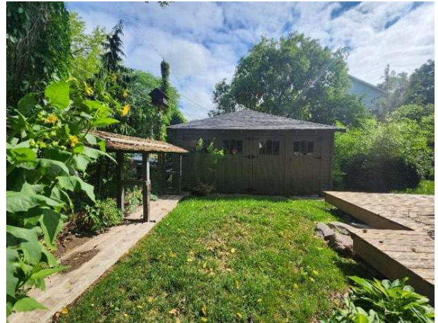
View of accessory building from the rear yard.
