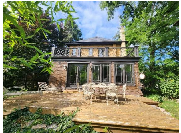
View of rear elevation of existing dwelling.
