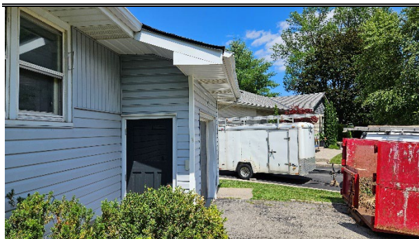
Existing garage projection looking towards abutting property at 245 Elmhurst Cres
