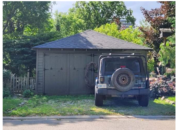
View of existing accessory building from Harris Crescent.
