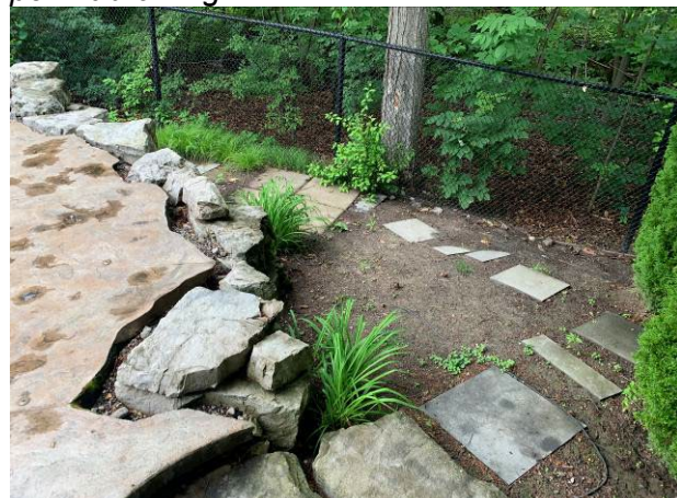
Retaining wall to be expanded into this corner of the property
