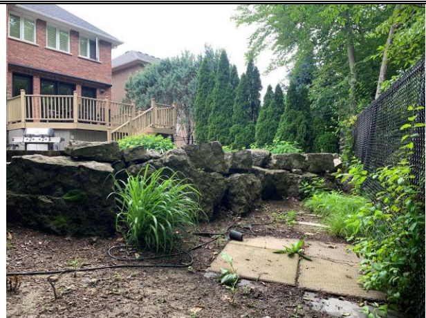
View along rear fenceline toward portion of retaining wall proposed to be removed
