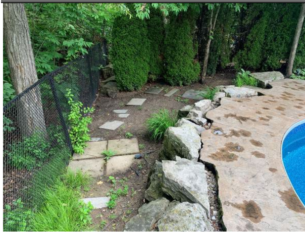
Alternate view of area targeted for retaining wall expansion
