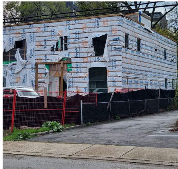
View of subject lands and constructed roof access from Bellview Street.
