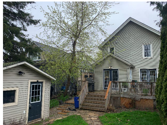
View of rear elevation of existing house
