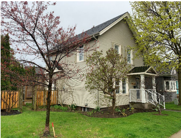
Front elevation and east elevation from corner of New Street and Delaware
