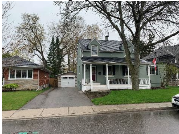
426 Delaware Avenue features a detached garage
