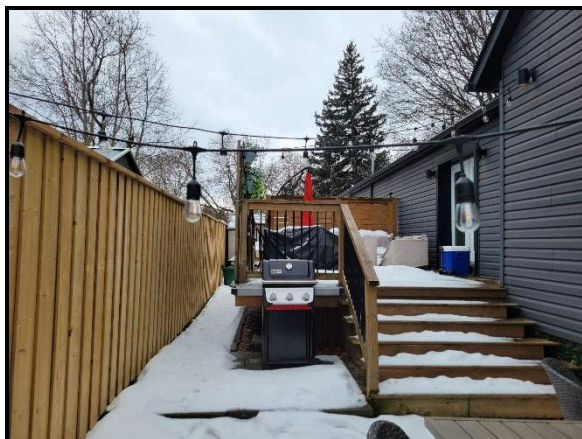
View of the existing deck (to be demolished) in the southeast side yard
