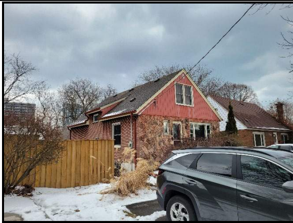
View of the abutting southerly property
