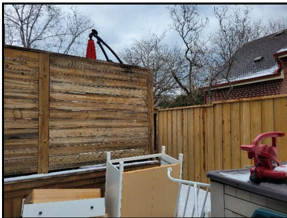
View of the existing deck in the southeast side yard
