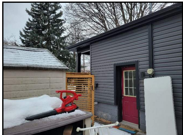
View from the southeast side yard towards the front gate
