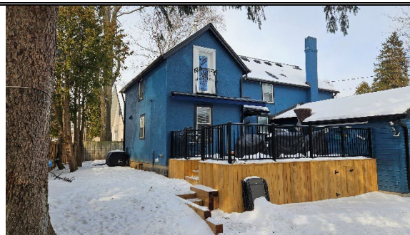
View of existing dwelling, from rear
