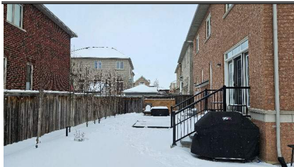
View of rear yard including swim spa, pool equipment and entry steps and landing
