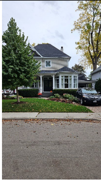
Nearby dwelling at 551 Hurd Avenue
