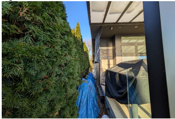
View of the existing southwest side yard
