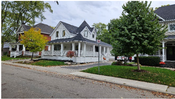
Nearby dwelling at 555 Hurd Avenue
