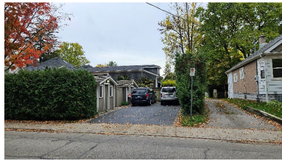
Nearby dwelling at 1406 Birch Avenue as well as accessory buildings at rear of 560 Hurd Avenue (at entrance to laneway on northerly side)
