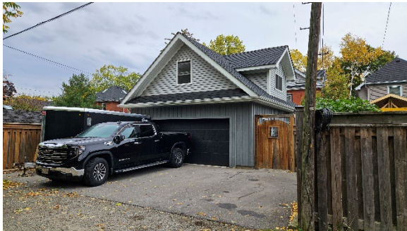
Two storey accessory building at 546 Hurd Avenue, accessible via rear laneway
