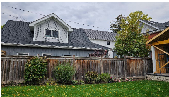
View from rear yard looking towards existing two storey accessory building at abutting property at 546 Hurd Avenue
