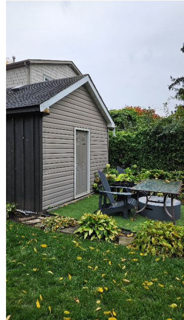
View of existing rear yard amenity space behind detached garage
