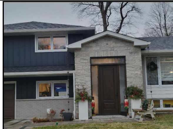
View of the porch enclosure
