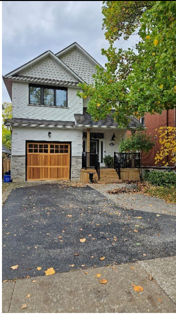
Nearby dwelling at 548 Hurd Avenue
