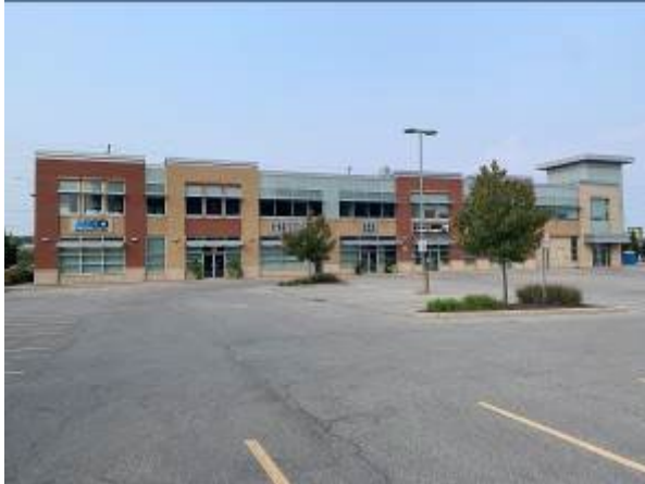
View of rear side of Building B
