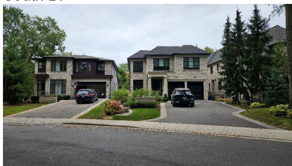
View of dwellings at 3034 and 3030 South Drive
