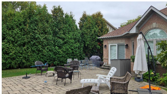
Rear of the dwelling at location of proposed addition (at sliding patio door)
