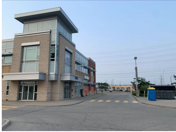
View of south end of Building A and main driveway entrance into the site from Appleby Line
