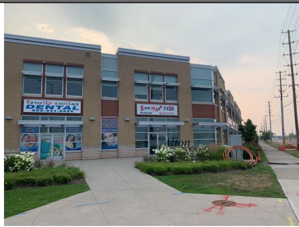
View of Building B looking north along Appleby Line
