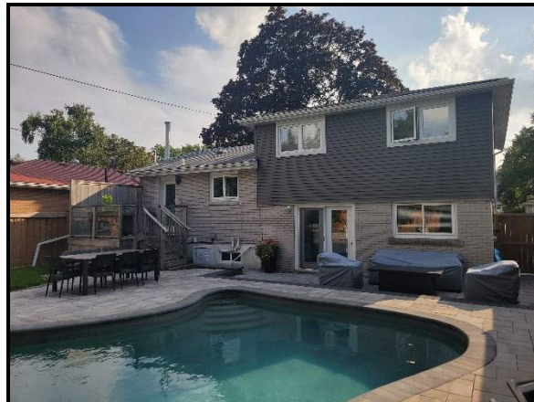
View of the dwelling from the rear
