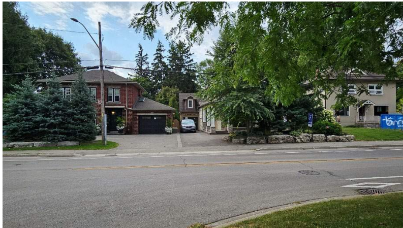
View of similar one-storey garage addition at 1020 North Shore Blvd E
