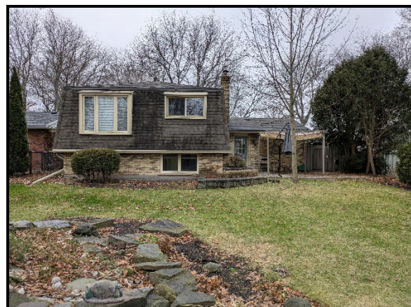
View of the rear of the existing house
