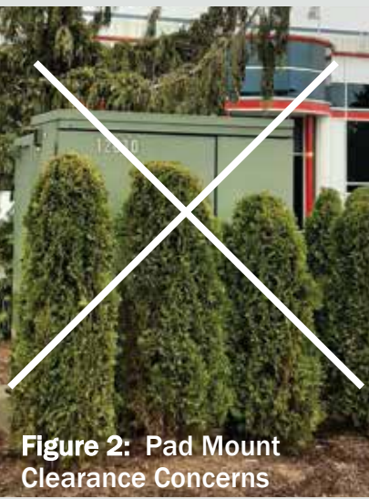
Figure 1: Clearances to Pad Mounted Equipment
