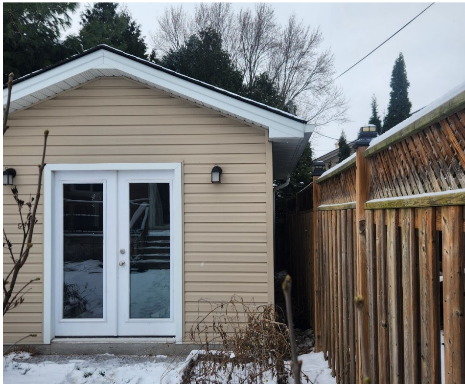
Close up of reduced south-east side yard setback.
