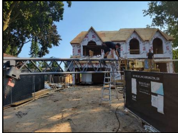
View of the abutting south easterly property
