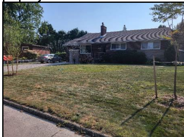
View of the northerly abutting dwelling
