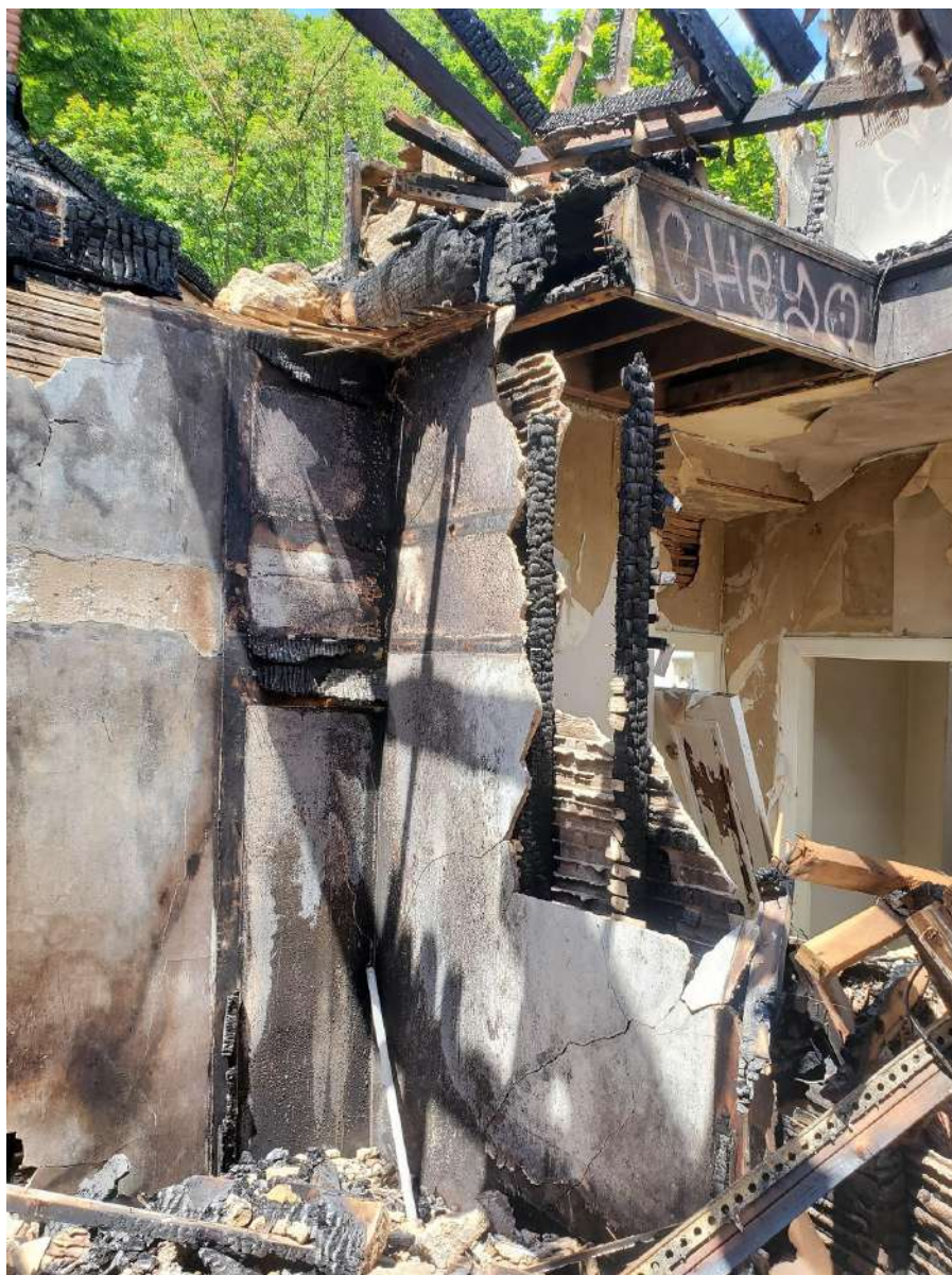
Figure 6: Condition of Much of the Remaining Interior Structure on South 2/3 of Building
