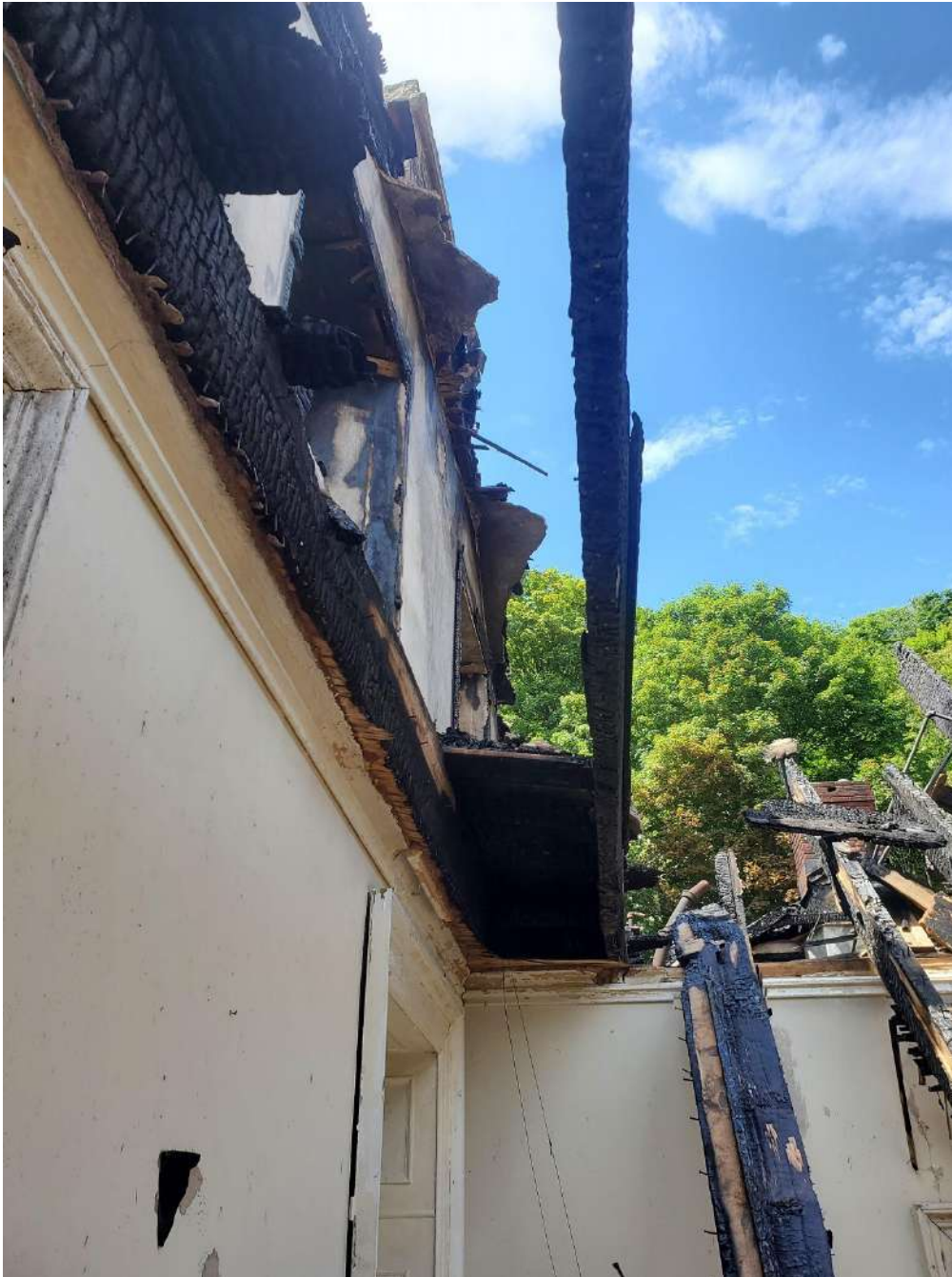
Figure 3: Typical Condition of 2 nd Floor and Roof Structure on South 2/3 of Building
