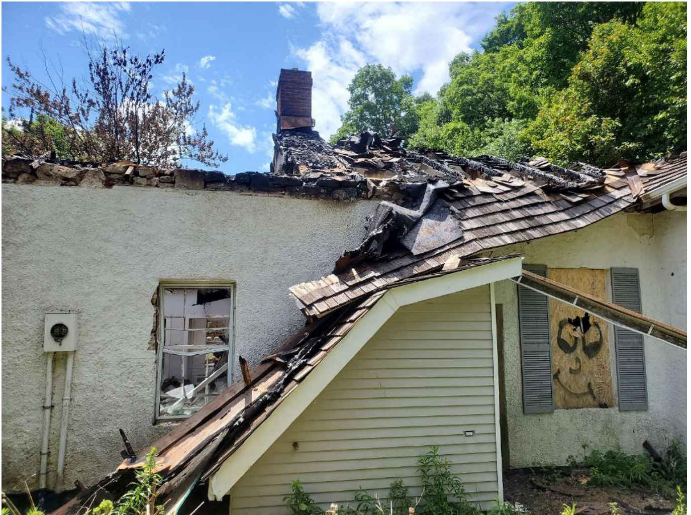
Figure 8: View From Outside of Building Looking West Showing Guttered Roof Structure to South and Fire Damage Extending Partially over North Portion of Building
