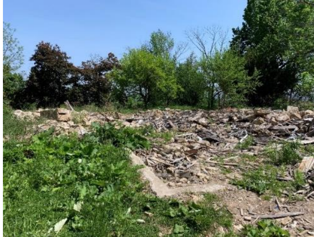
Main House Current Condition (2022).
