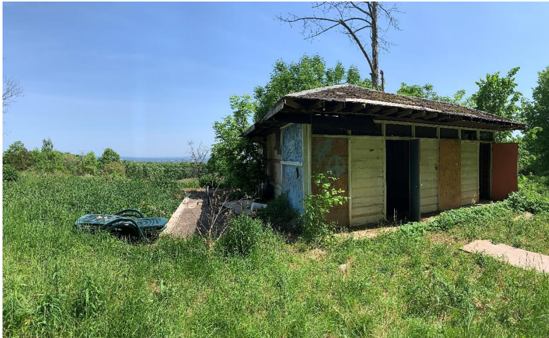
Cabana Building (No heritage significance)
