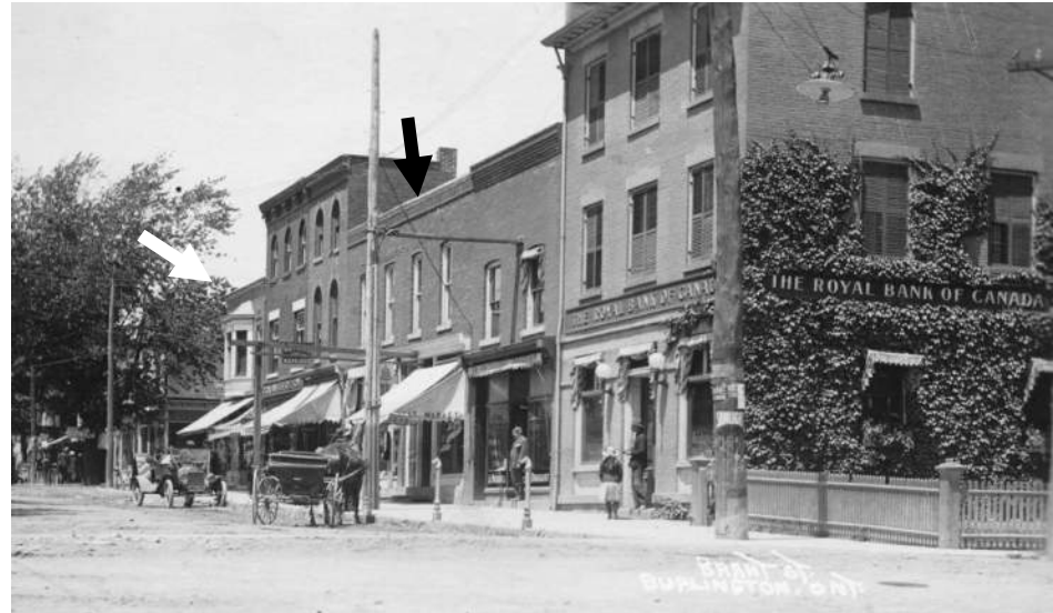
1914 post card of Brant Street looking north from what was then Water Street. From "The Prints of Burlington."
