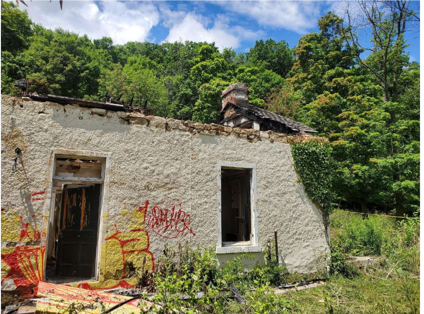
Figure 7: View From Outside of Building Looking North
