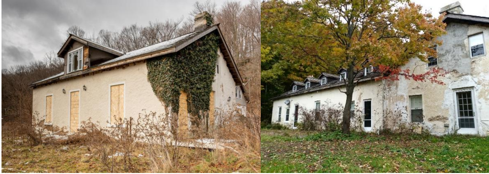
South (front) elevation and west (side) elevation before the fire.
