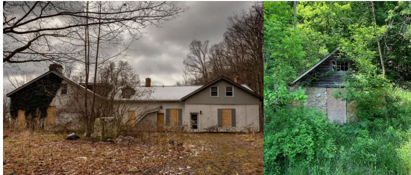
Side (east) elevation before the fire & the Woodhill Ice House (2022).
