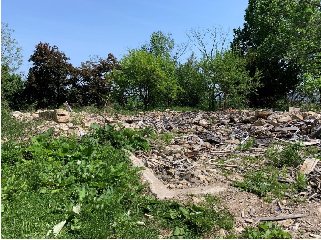
Demolished main house after the fire -View south towards Burlington Bay
